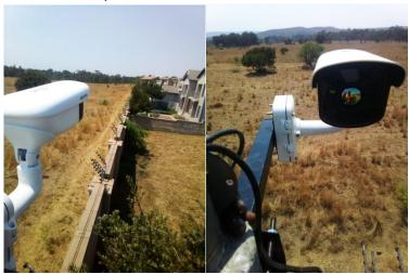
Hikvision ANPR Cameras have also been installed at the site's three entrance and exit points, providing an overhead view of vehicles coming into and leaving the estate 24 hours a day. These cameras offer license plate recognition technology to ensure that only authorized vehicles are admitted.
