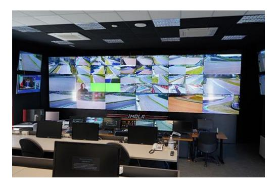
"In this regard, our proposal consists a 4K video system with fixed and motorized cameras all along the circuit, connected via Dahua switches [2x PFS5924-24X and 1x PFS4218-16ET-240] to an appropriately sized network infrastructure to avoid latency, while our customized DSS server [DSS4004-S2] manages real-time records and instant playback inside the control room," explains Diego Schiraldi, Area Sales Manager of Emilia-Romagna region of Dahua Technology Italy.
