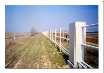
Each zone of the Radiocontact Leaky Feeder Perimeter Fence Movement Detection System covers 100m with a resolution of 50m to accommodate for suitable depth of field coverage support with CCTV surveillance. A typical zone installation is shown bellow.
