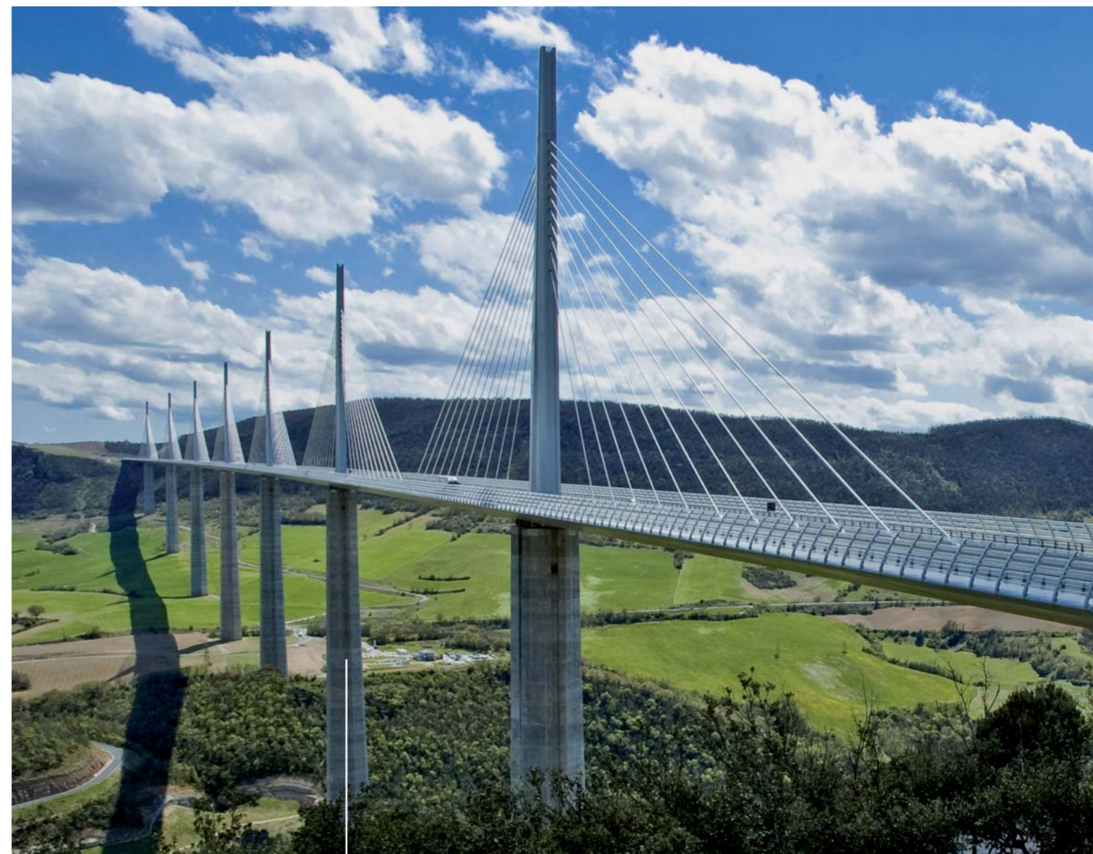
Millau viaduct, France | traffic monitoring | toll supervision Further references at www.geutebrueck.com
