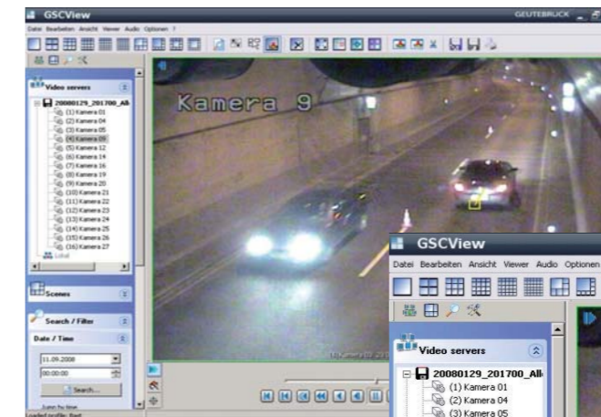
Application: Tunnel security
