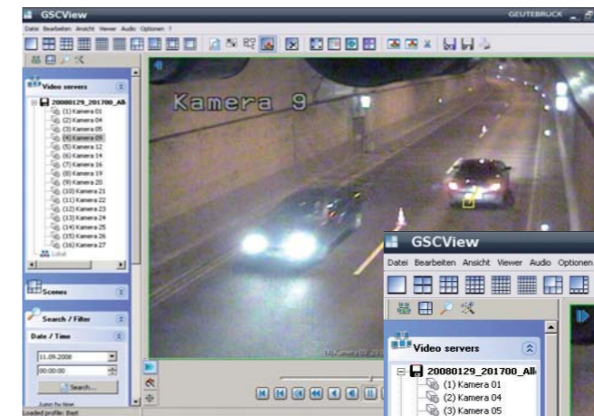
Application: Tunnel security
