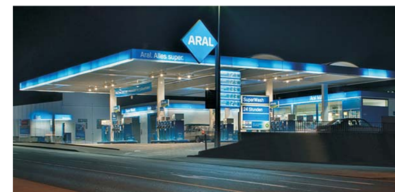
Filling station security | pump monitoring | shop monitoring | cashier system recording
