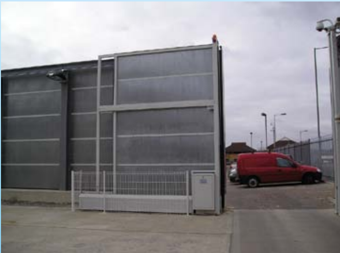
Bespoke LoTracker Cantilevered Gate 5m high x 3m wide, with special acoustic sheet infill.
