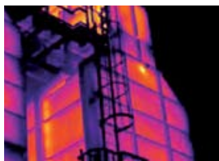
Petrochemical & chemical industries
